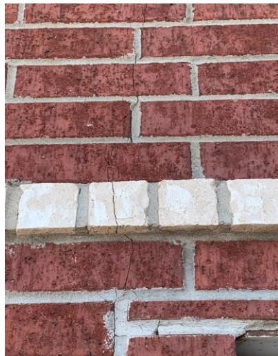
Cracking Brick
