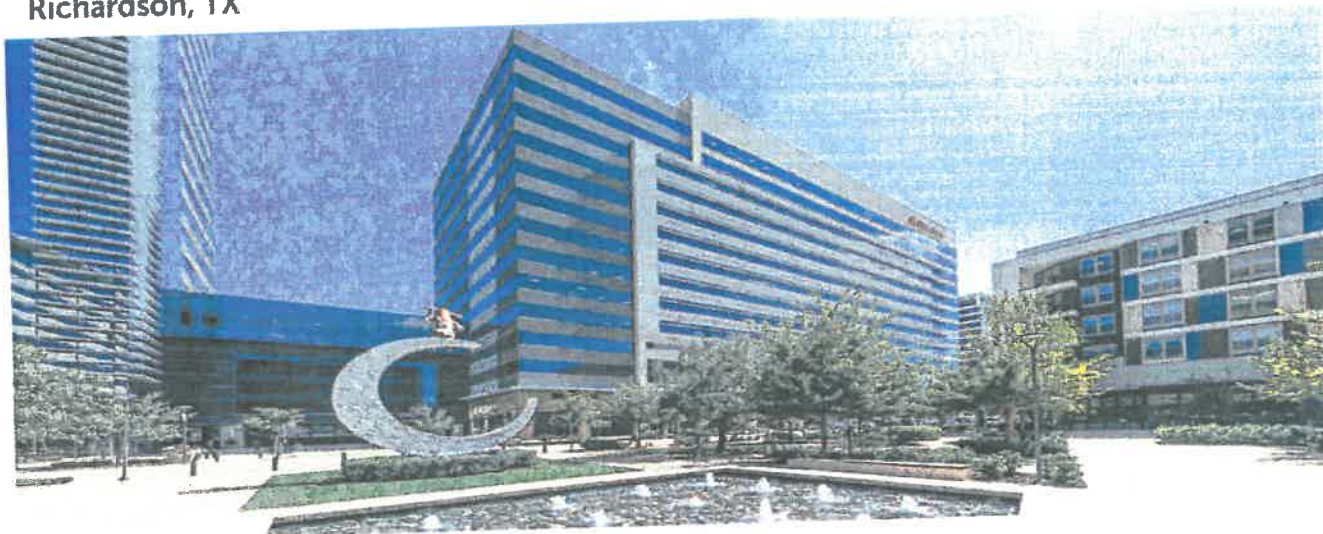
State Farm Headquarters Richardson, TX
