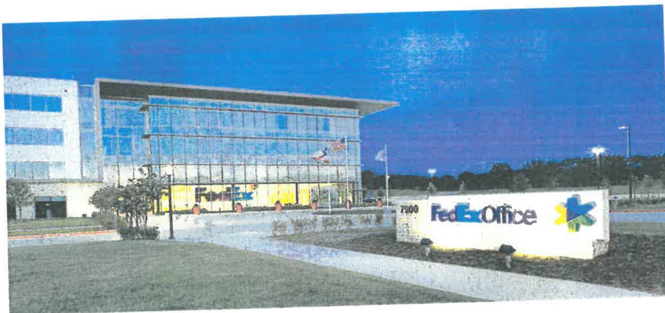
FedEx Office Headquarters Plano, TX
