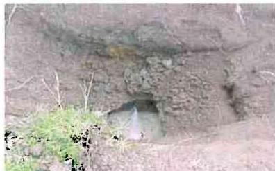
Some leaks cannot be seen from ground level. In this example, the soil above this leak is bone dry.
