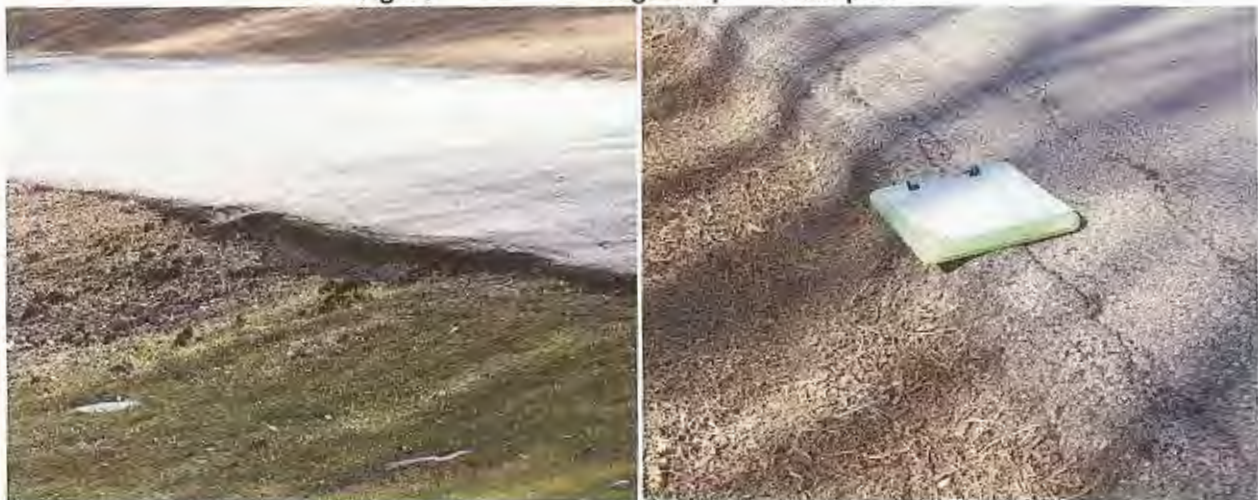
Figure 4: Pavement Edge Drop Off Examples
