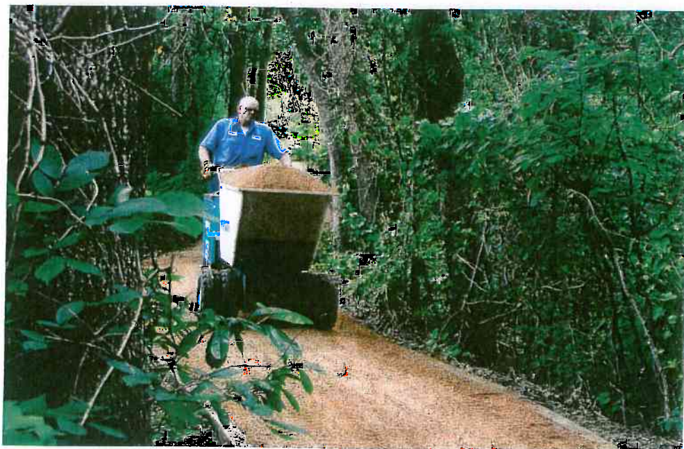
Method of placing material and initial compaction
