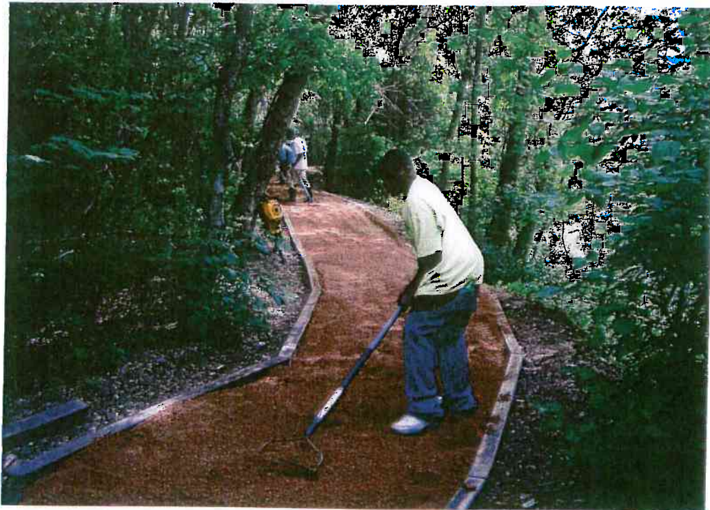
Deposed granite is placed and leveled
